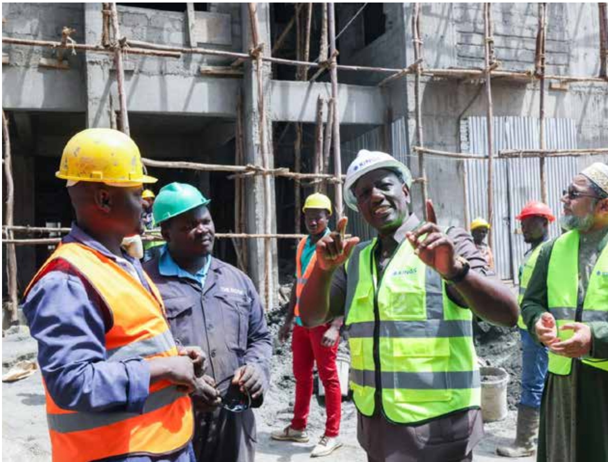
President William Ruto during a site visit at the Kings Boma Estate, an affordable housing project in Ruiru town, Kiambu county.
