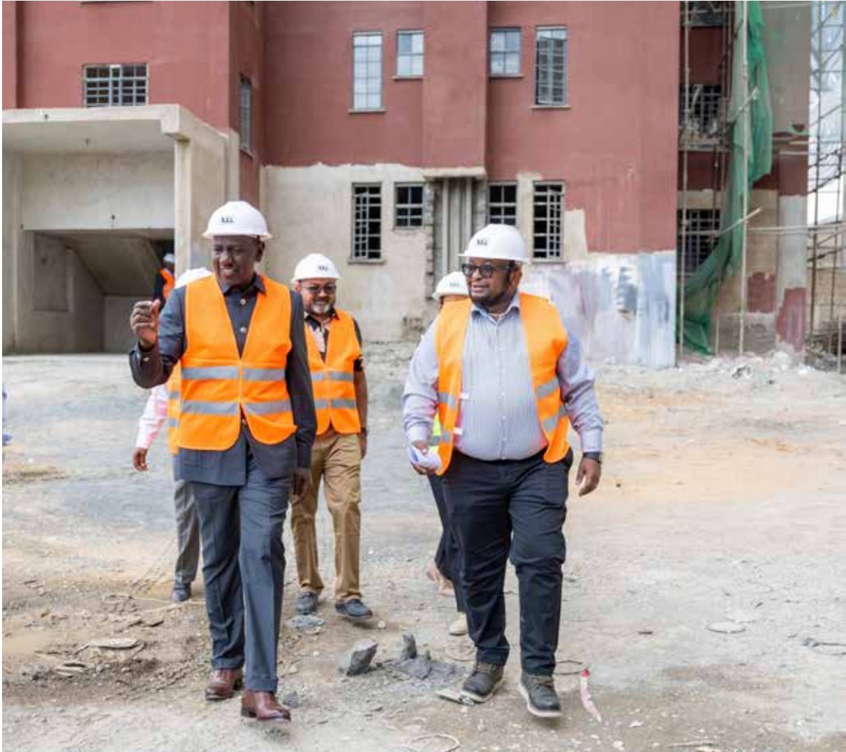
President William Ruto inspecting construction of affordable housing units.
